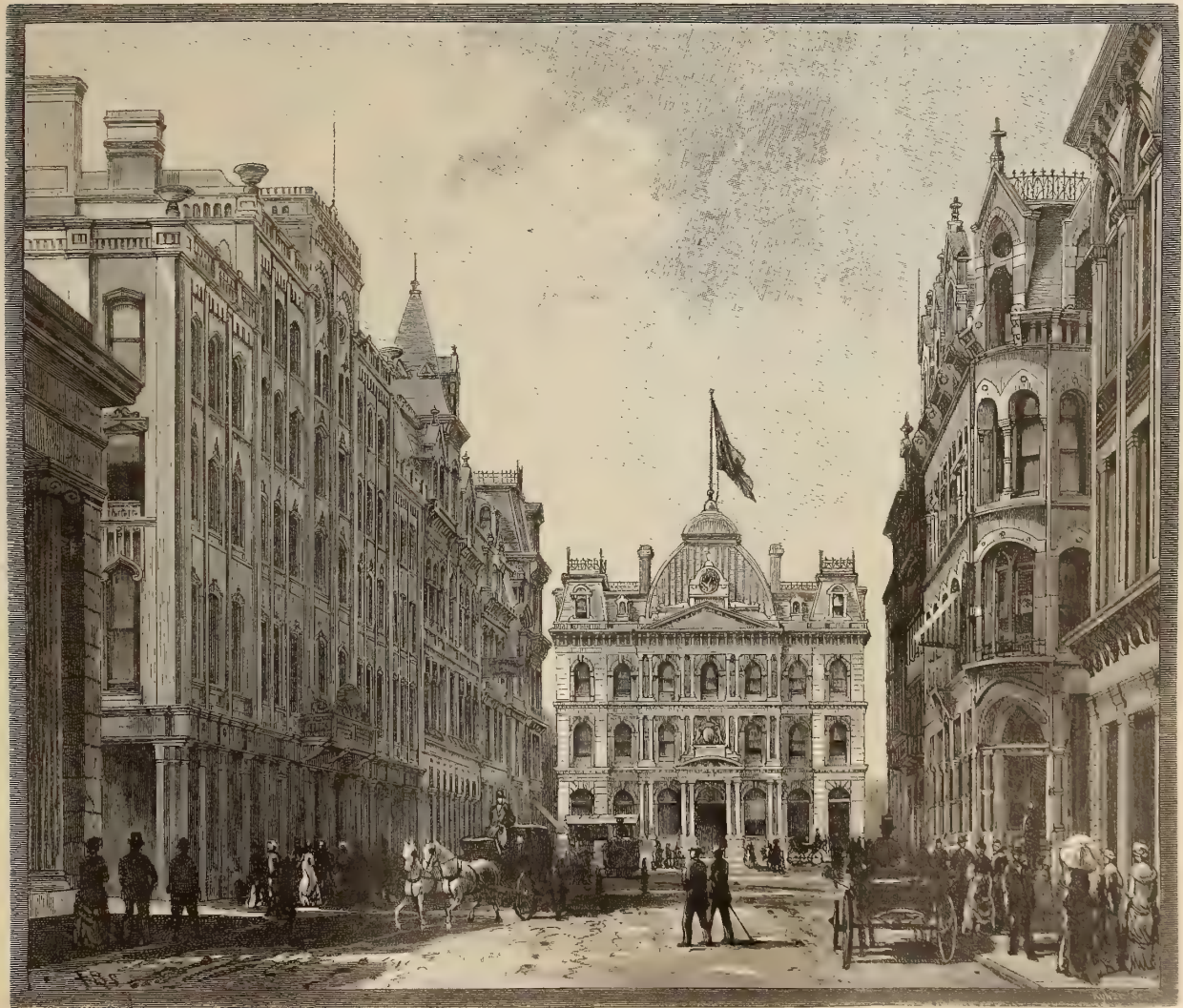
TORONTO STREET, AND POST OFFICE.
